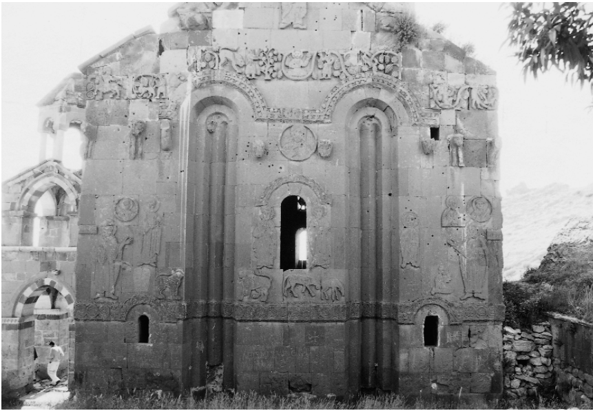
4.24 East façade, Church of the Holy Cross, Aght'amar
